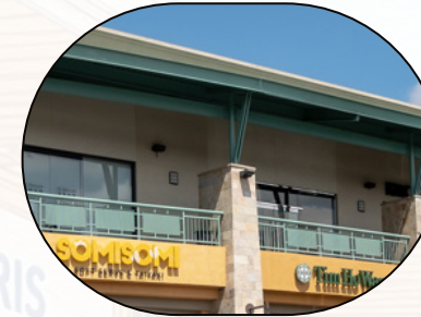
Continuous Building Overhang
