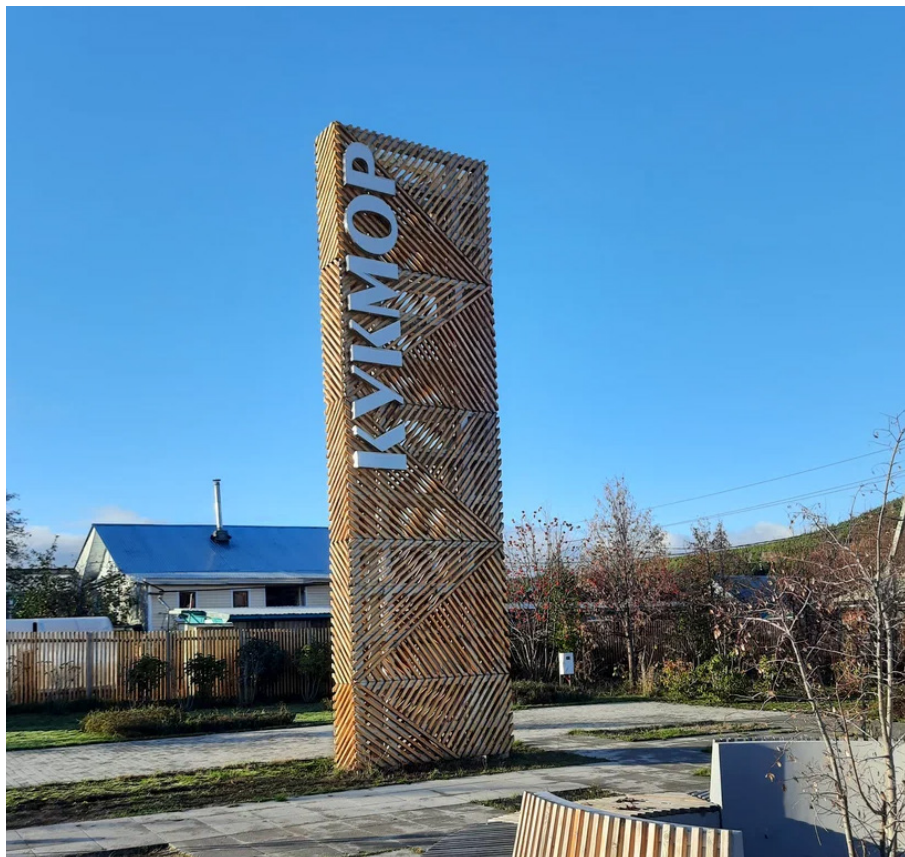
Pylon sign constructed of wood slats with integrated vertical lettering and decorative geometric screening.
