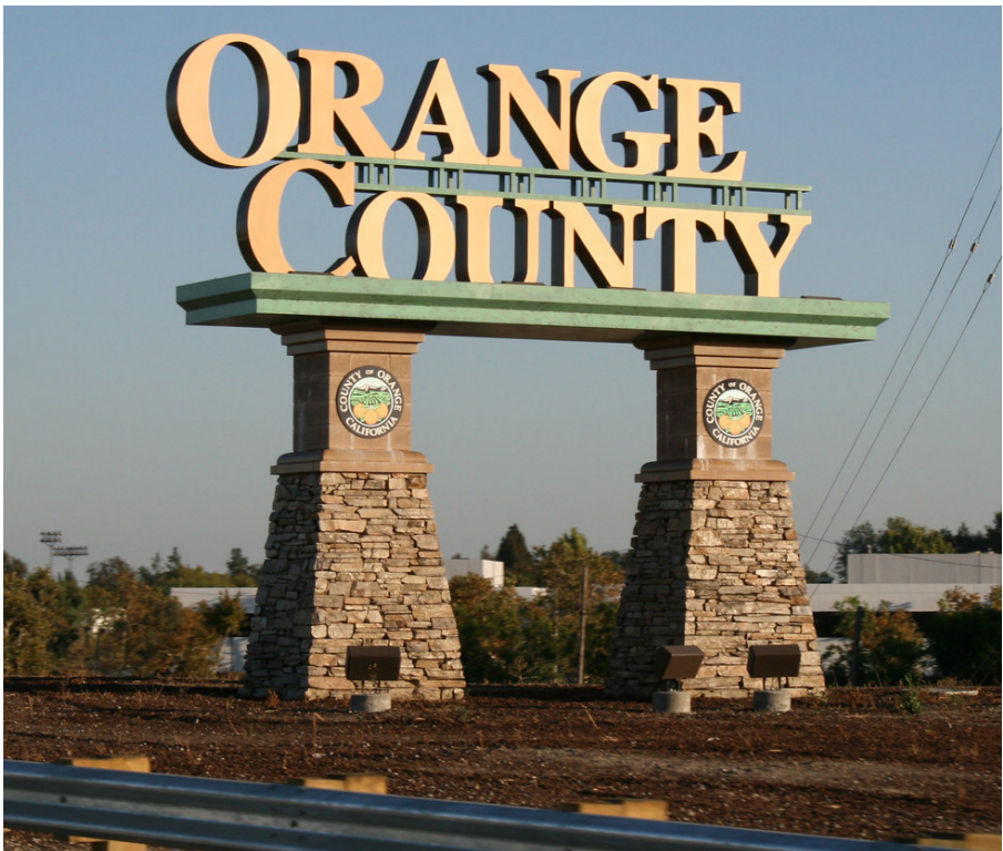
Large-scale monument sign featuring dimensional lettering and architectural supports.
