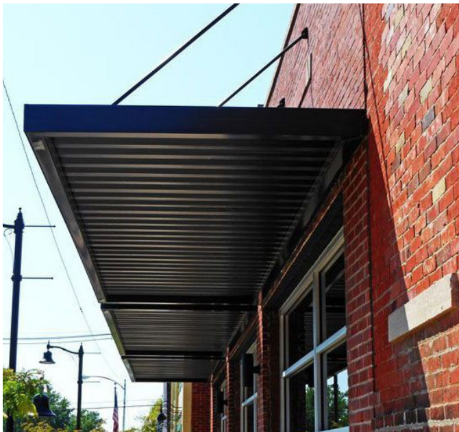
Cantilevered Metal Canopy
