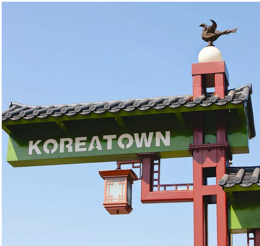
Cantilevered gateway featuring traditional roof forms, decorative lanterns, and cultural detailing.
