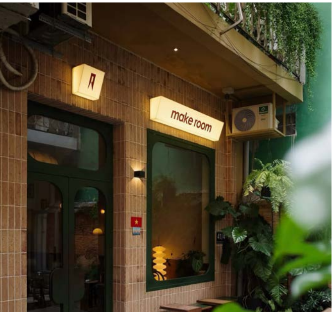
Ceramic tile cladding facade complemented with dark painted metal framing system.
