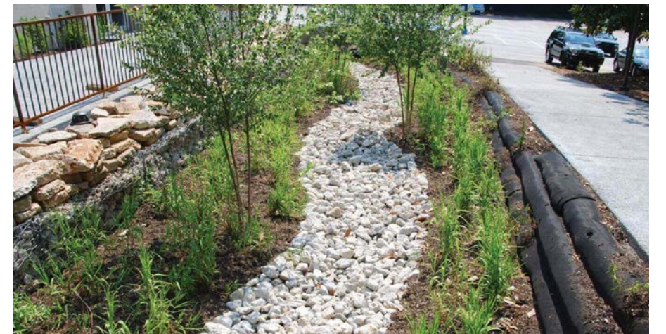
Vegetated bioswale capturing and filtering stormwater runoff along sidewalk.
